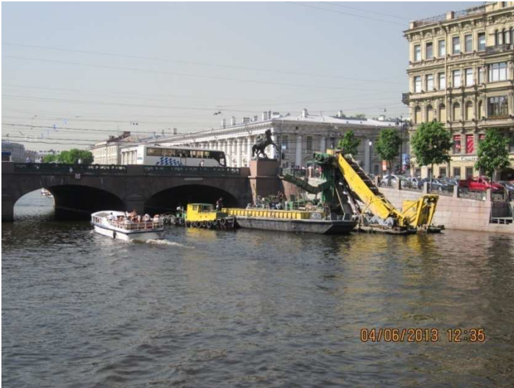
Work on clearing the bed of the river of Fontanka river section from Scherbakov lane to bridge Belinsky. the year 2013
